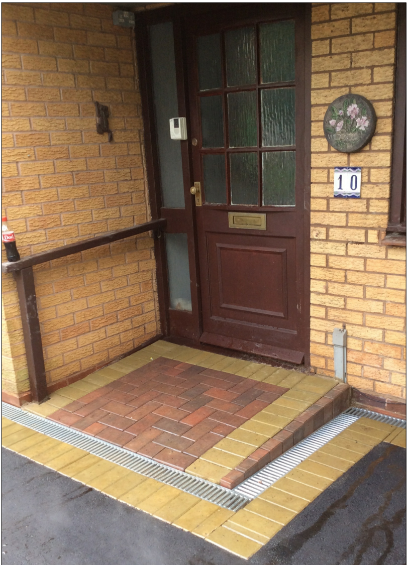
Sample: Access ramp
