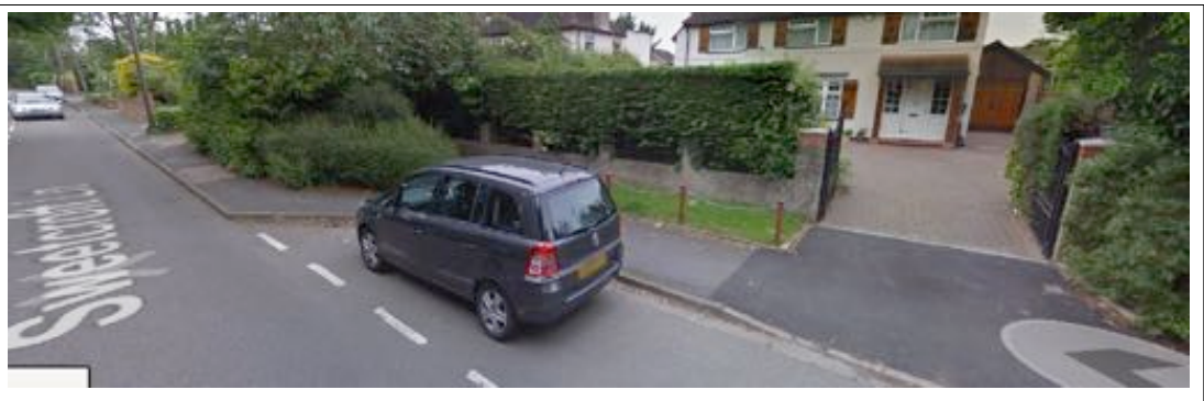
No.10 Sweetcroft Lane - Brick wall with piers and box hedging infill
