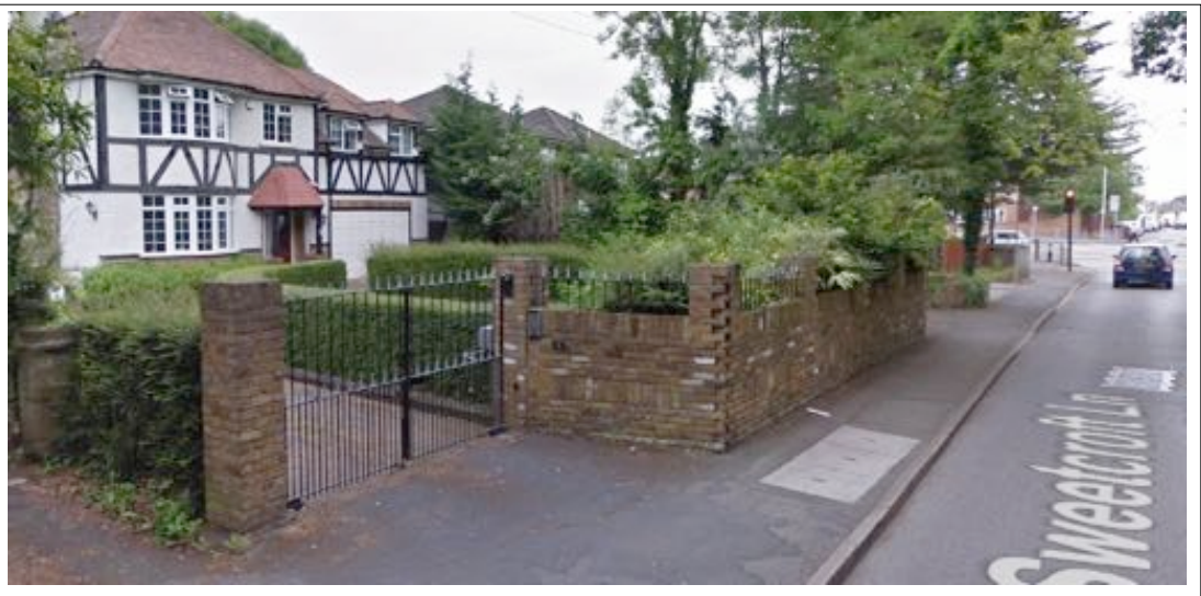
No.4 Sweetcroft Lane - Brick wall and piers with ironwork infill
