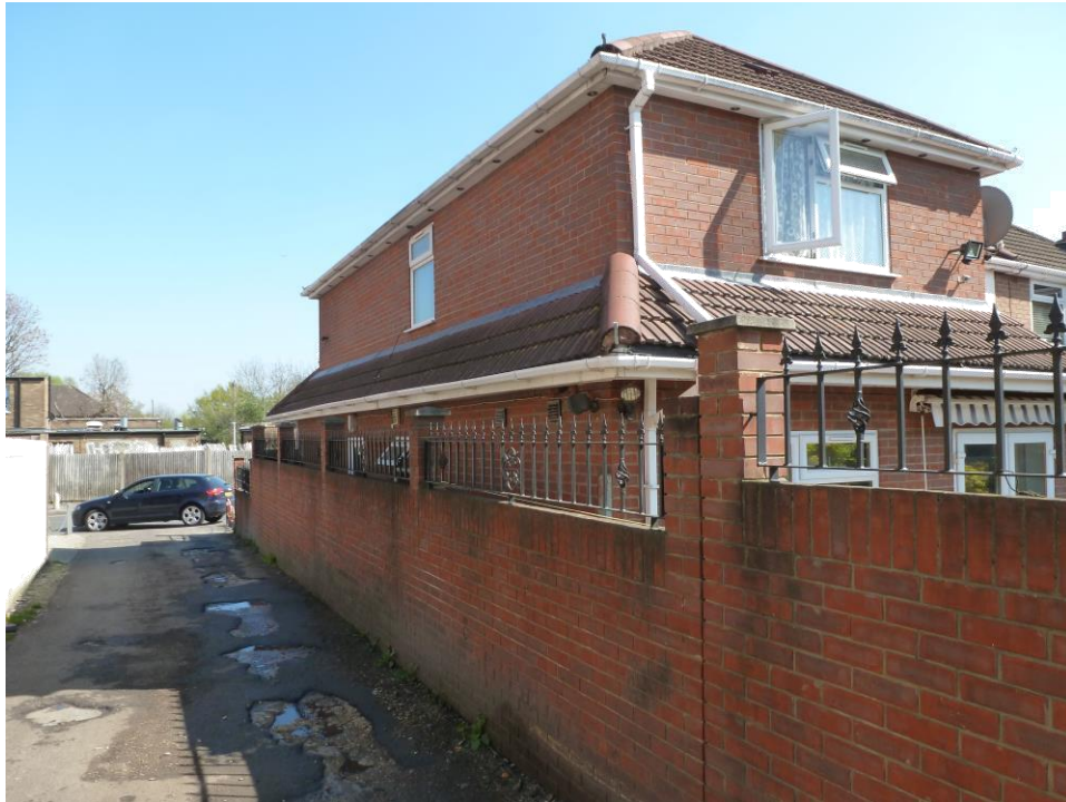
Fig. 4. Rear of no. 1 Roseville Road from alleyway
