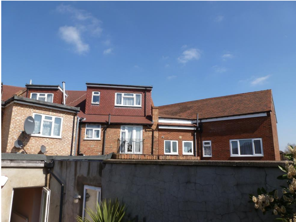
Fig. 6. View of rear of nos. 169, 171 and 171b North Hyde Road
