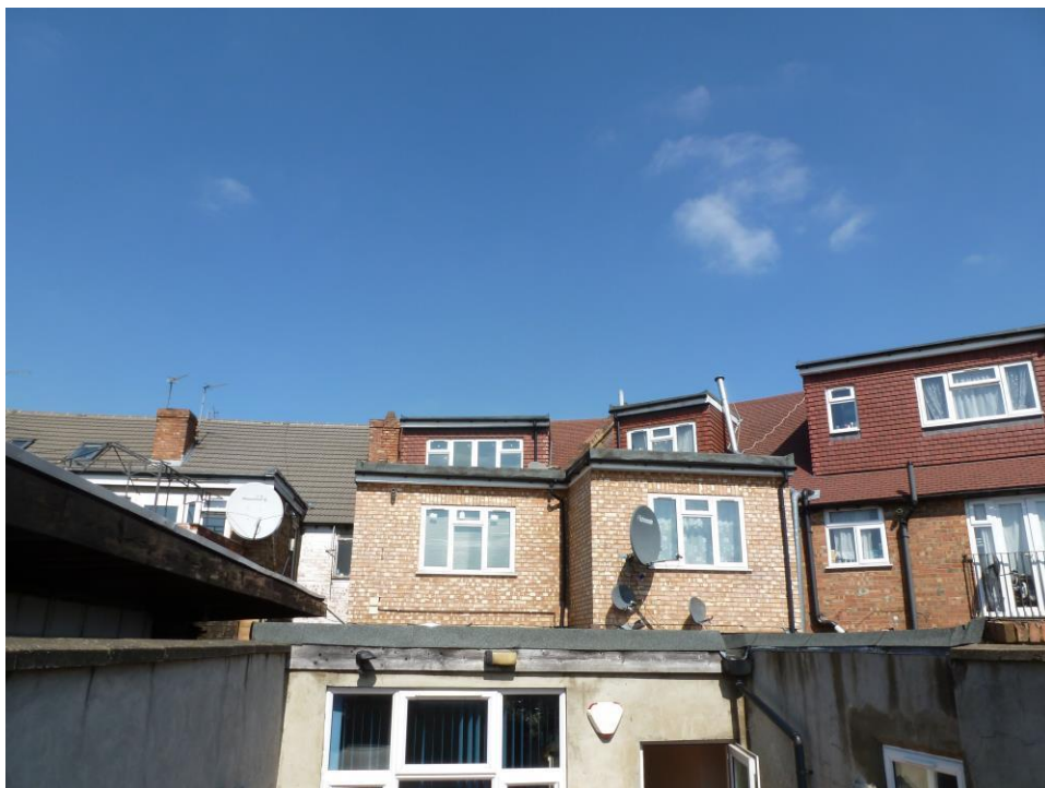
Fig. 5. View of rear of nos. 165, 167, 169 and 171 North Hyde Road
