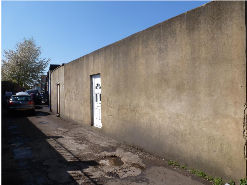
Fig. 11. Existing boundary to rear alleyway
