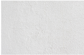
White render to finish external elevations
