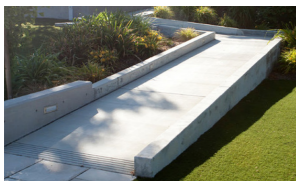
Ramped approach to the main entrance with gradient 1:12
