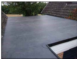
PROPOSED EPDM FLAT ROOF - BLACK EPDM RUBBER ROOFING MEMBRANE
