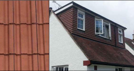
RED CONCRETE TILES TO PROVIDES A LOW PROFILE ROOF AND TO MATCH EXISTING NEIGHBOURS' ROOFS ON GREEN WALK.
