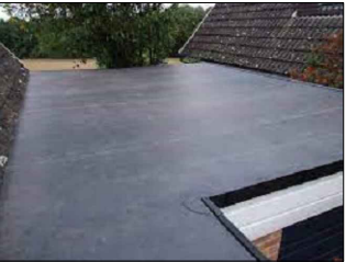
PROPOSED EPDM FLAT ROOF - BLACK EPDM RUBBER ROOFING MEMBRANE BY RUBBER ROOFING DIRECT
