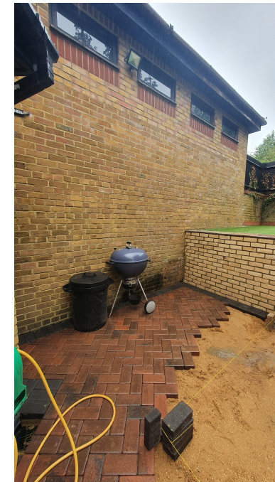
Double garage - north side (1 owned by 8 Jacks Lane and 1 owned by 9 Jacks Lane)
