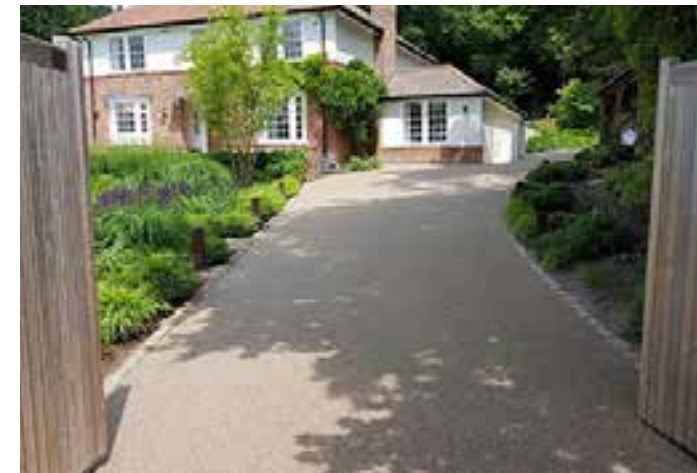
Driveway - Resin Bound gravel - The Resin Mill - Colour Cappucino Fall of 1:75 sloping away from garage door
