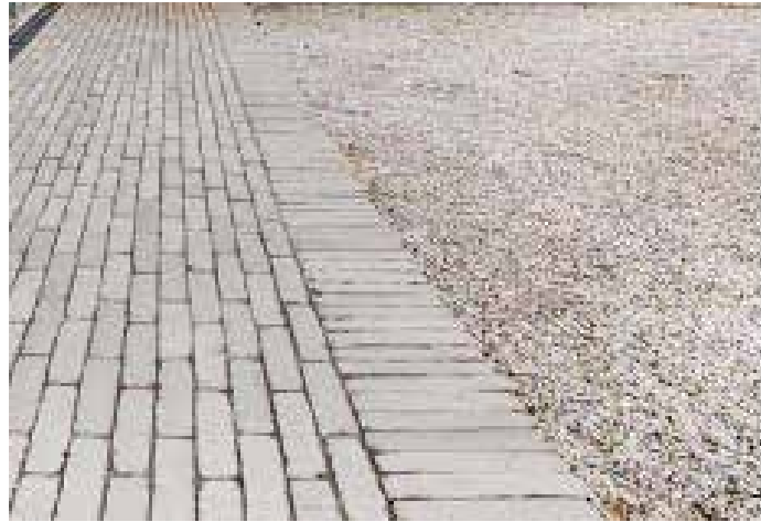
Clay pavers laid in stretcher bond with 2-3mm nominal joints filled with jointing sand and min slope of 1-2% Vande Moortel SeptimA Olive Paver edging supported by sand cement - Slot drains where required
