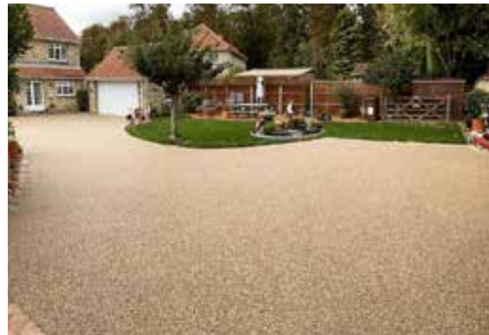
Driveway - Resin Bound gravel - The Resin Mill - Colour Cappucino Fall of 1:75 sloping away from garage door
