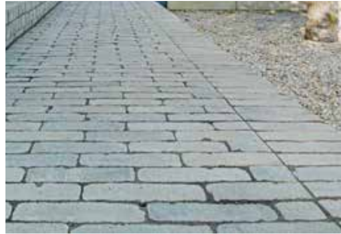
Clay pavers laid in stretcher bond with 2-3mm nominal joints filled with jointing sand and min slope of 1-2% Vande Moortel SeptimA Olive Paver edging supported by sand cement - Slot drains where required
