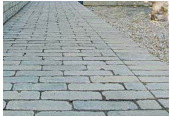
Clay pavers laid in stretcher bond with 2-3mm nominal joints filled with jointing sand and min slope of 1-2% Vande Moortel SeptimA Olive Paver edging supported by sand cement - Slot drains where required
