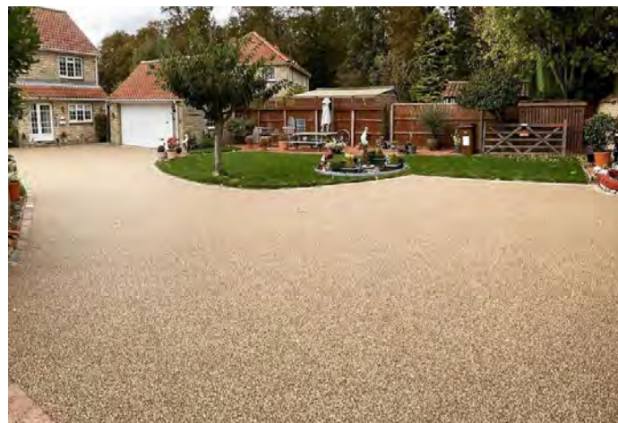
Driveway - Resin Bound gravel - The Resin Mill - Colour Cappuccino Fall of 1:75 sloping away from garage door
