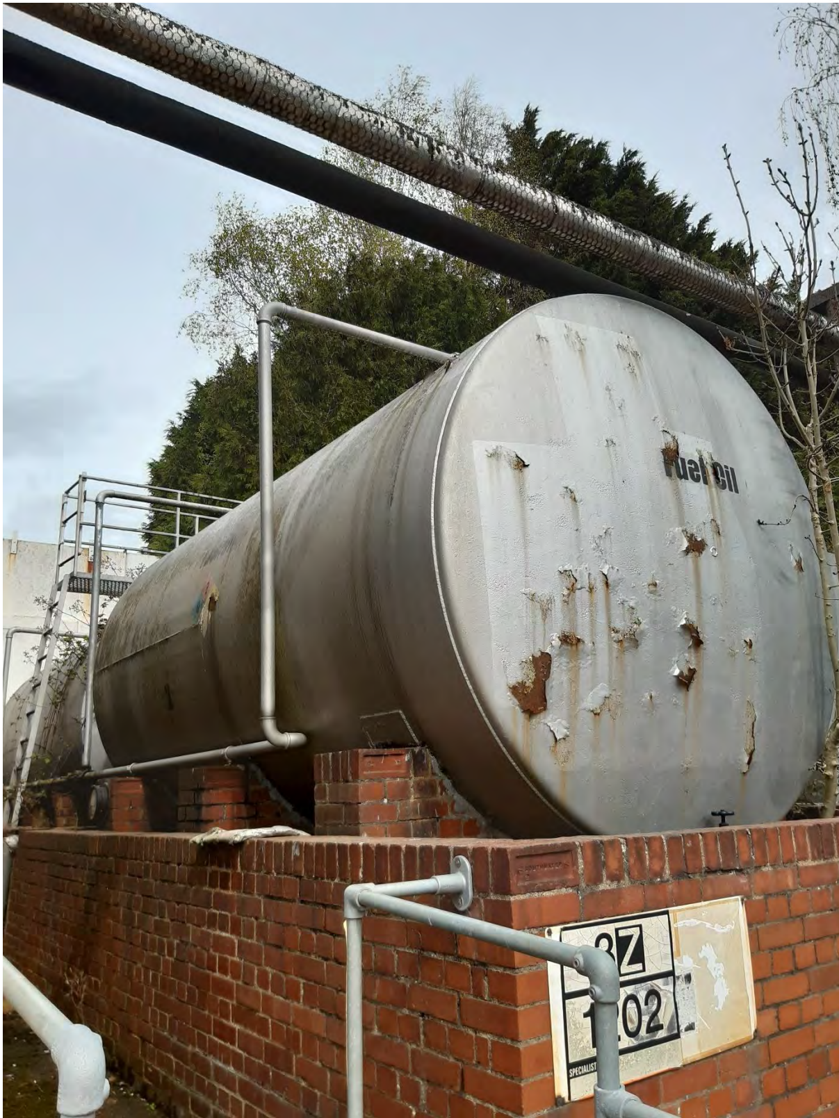
Plate 9: View towards the north-east, taken from the eastern area of the site. Showing large cylindrical above ground fuel storage tanks within brickwork bund.
