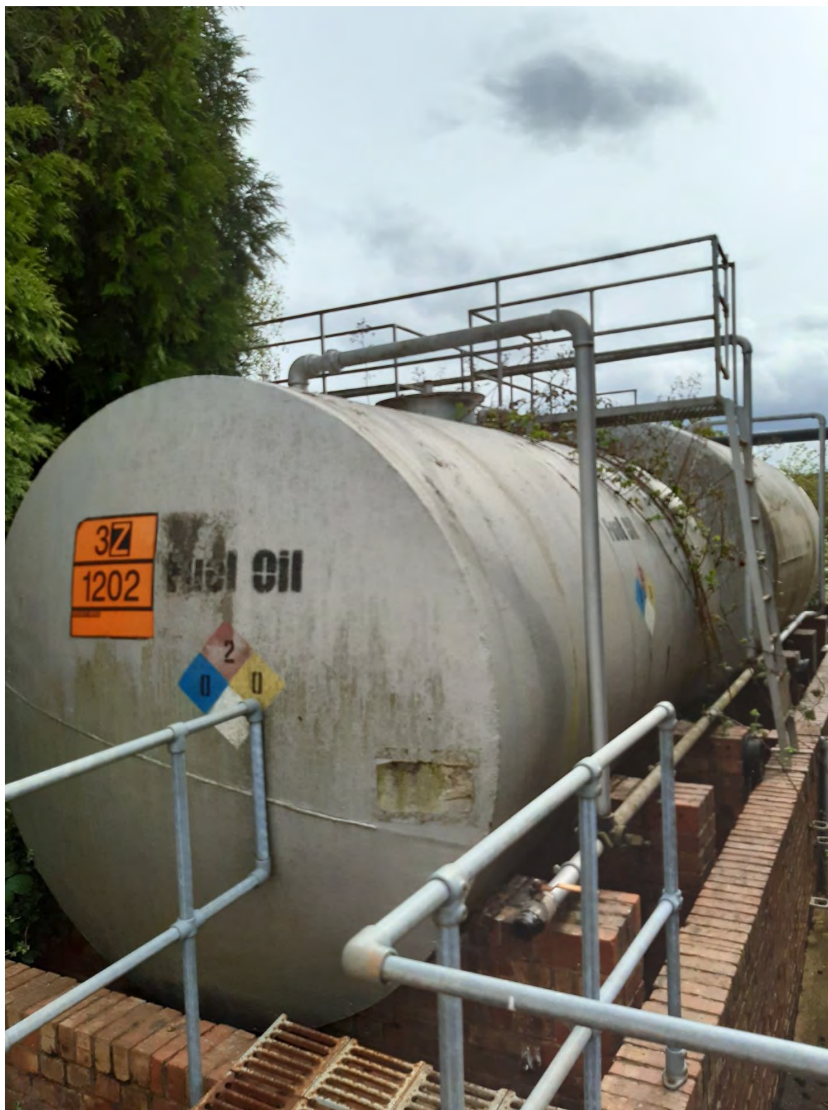
Plate 10: View towards the south-east, taken from the eastern area of the site. Showing large cylindrical above ground fuel storage tanks within brickwork bund.
