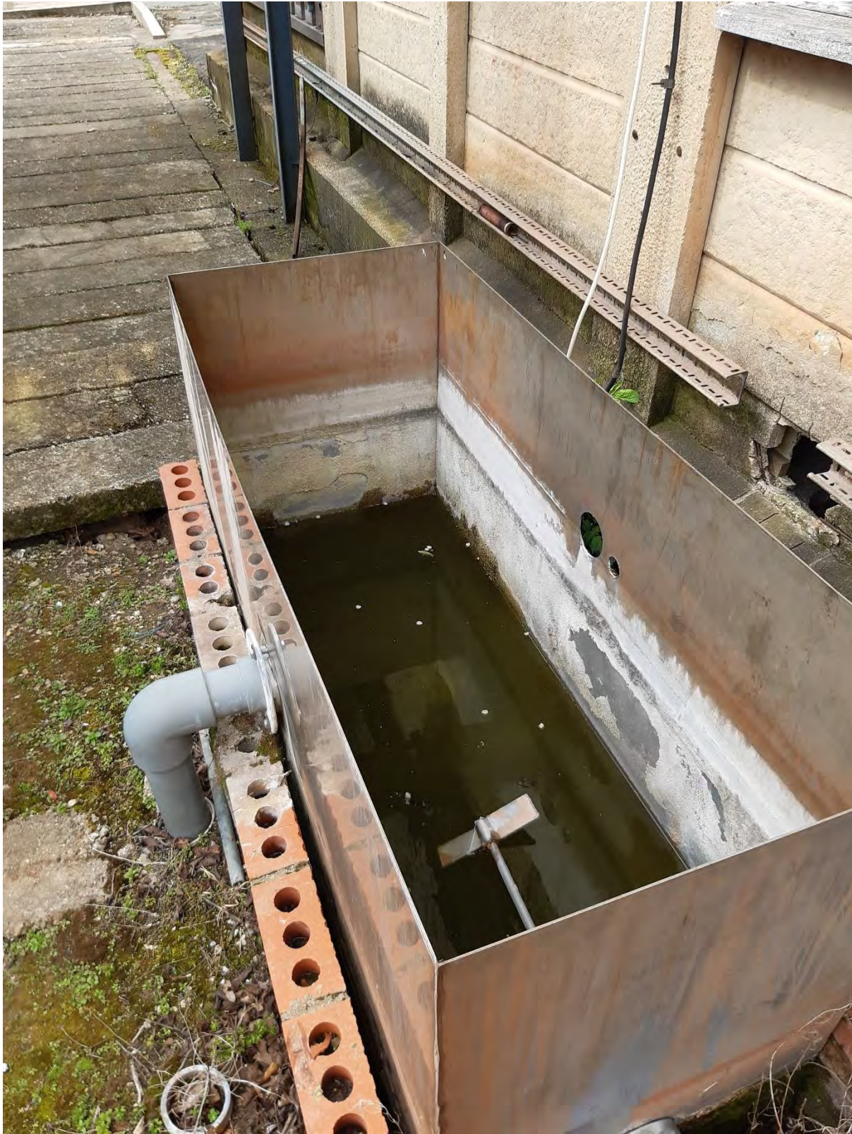
Plate 8: View towards the north-west, taken from the south-eastern area of the site. Showing decommissioned rectangular above ground storage tank adjacent to building 28.
