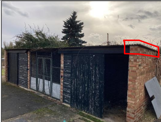
Figure H. B7, east elevation. Gap between roof and wall top indicated
