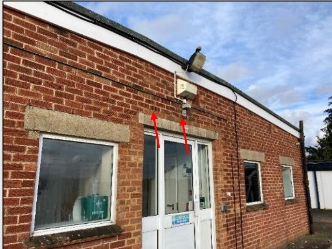
Figure R. B17, south elevation. Gaps above lintel indicated
