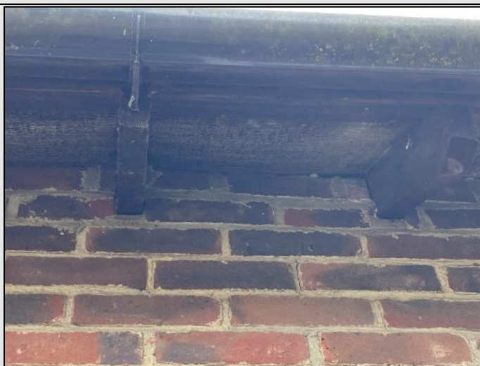
Figure G. B6, north elevation. Photo showing overhanging eaves with gap at wall top providing potential ingress to loft
