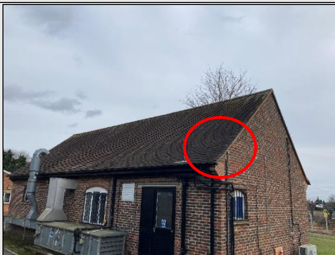
Figure F. B5, north-west elevation. Lifted roof tiles and gaps in roof verge mortar indicated
