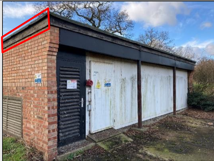
Figure Q. B16, southwest elevation. Fascia with gap indicated.
