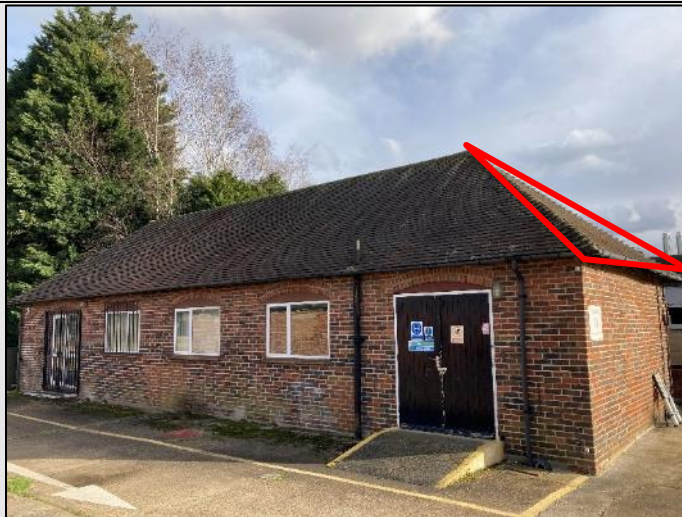
Figure K. B10, north elevation, lifted bonnet tiles highlighted
