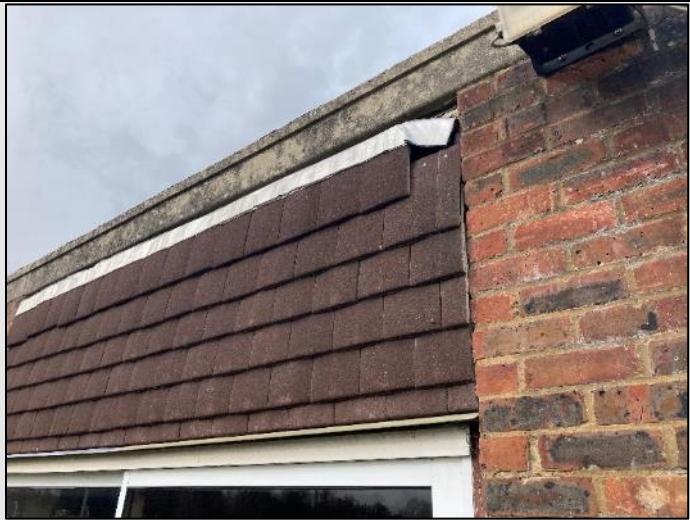
Figure B. B1 missing hanging tiles and lifted lead flashing, southeast elevation
