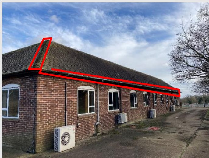
Figure P. B15, east elevation. Gaps at eaves and lifted bonnet tiles indicated
