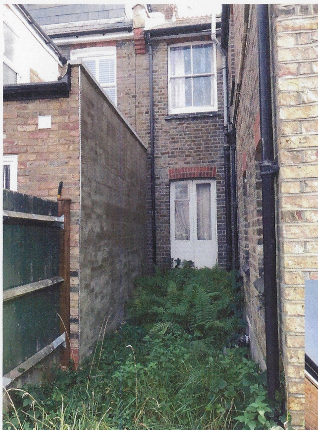
Photo 1 - Rear elevation of 14 Rofant Road, looking onto 16 Rofant Road with 2.9m eaves.
