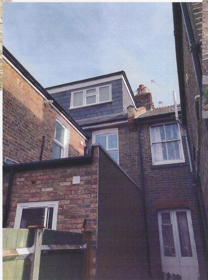
Photo 2 - Rear elevation of 16 Rofant Road, side extension and loft extension.
