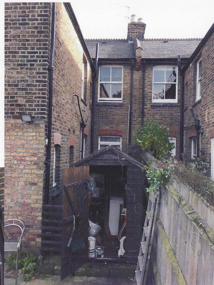
Photo 3 - Rear elevation of 12 and 10 Rofant Rd
