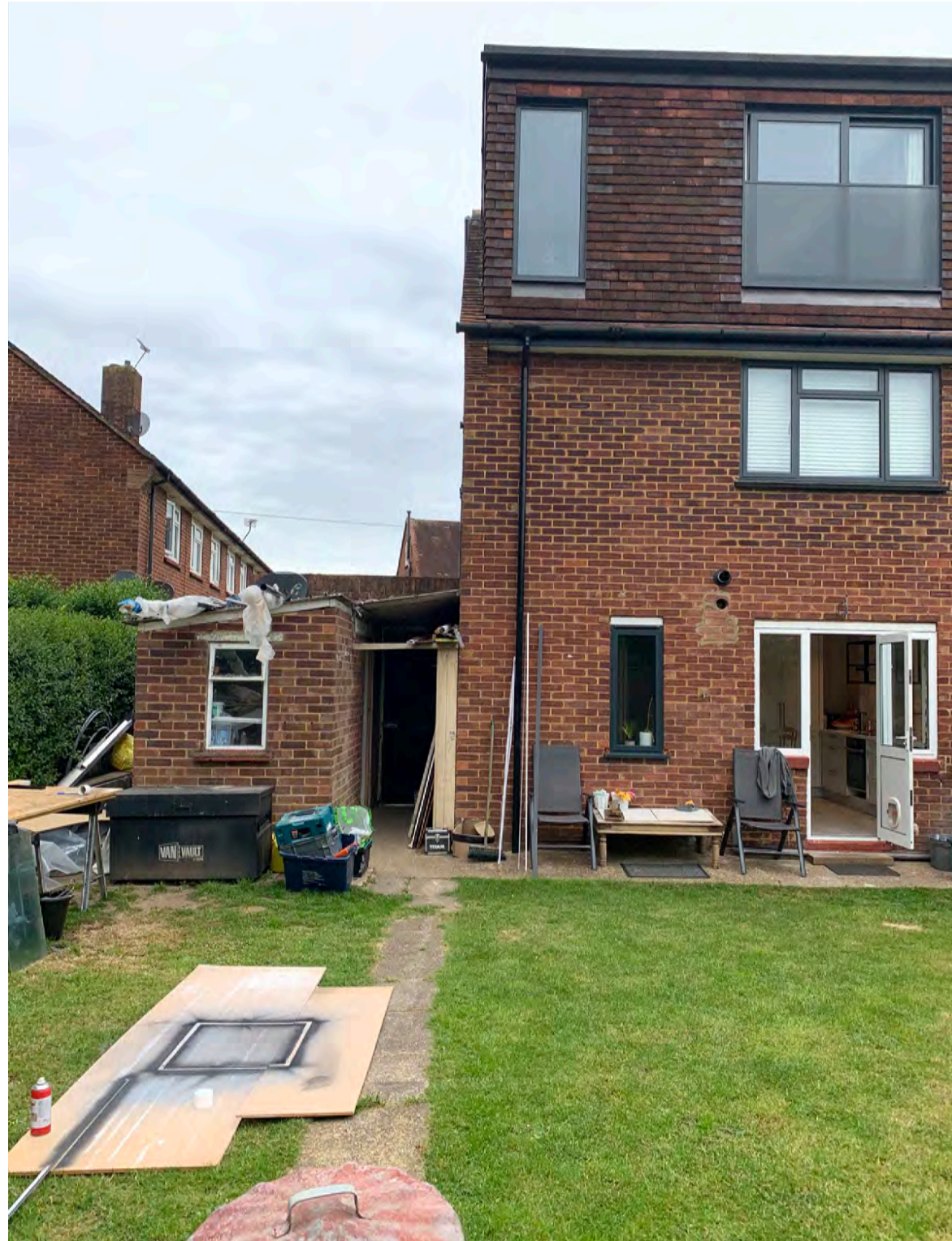
10. View of the rear showing existitng hedge and outdoor buildingt to be demolished.
