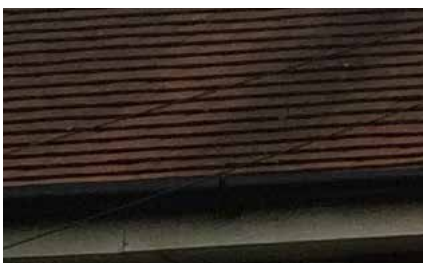
Existing Tile Roof
