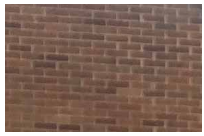
Existing Brick work
