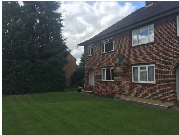
House adjacent Access Road- Southbourne Road
