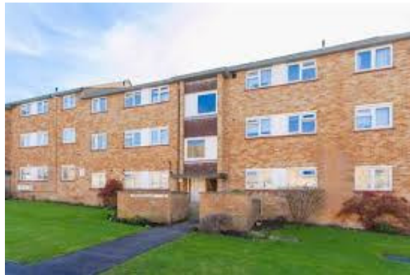
Three storey Flats – North of Site
