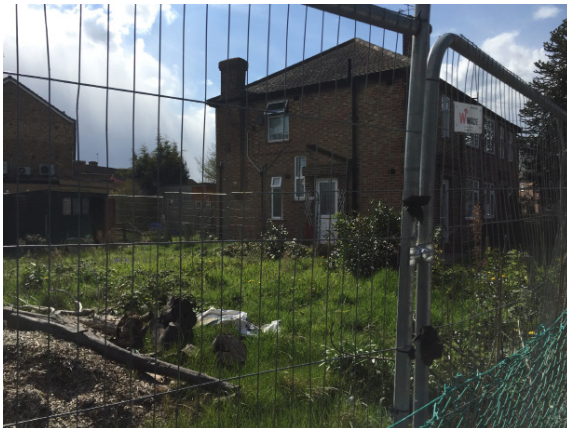
Fig.13. Existing frontage to Botwell Crescent.
