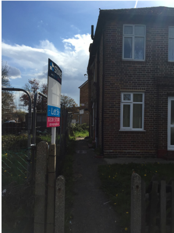
Fig.8. Existing boundary to 13 Botwell Crescent.
