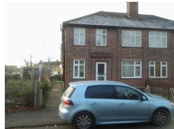
Fig.10. 1-3 Botwell Crescent primary elevation.
