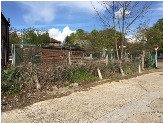
View of the existing site from Judge Heath Lane.
