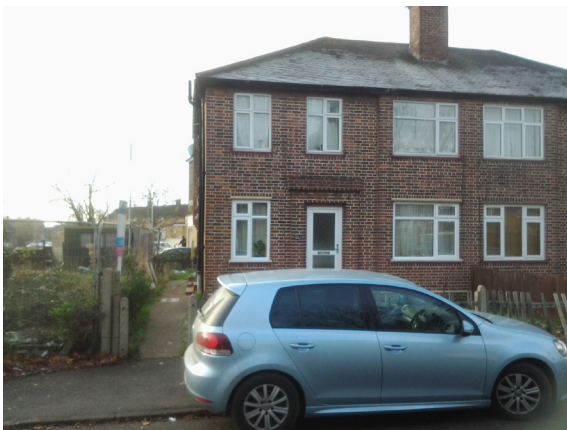
1 3 Botwell Crescent primary elevation.
