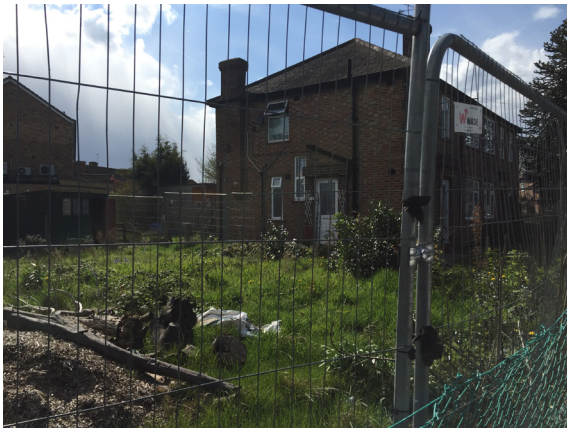
Existing frontage to Botwell Crescent.
