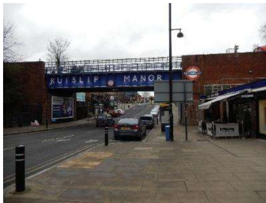
View of railway bridge from Victoria Road, from the north (left, facing) and south (right)
