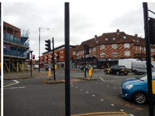
View of north-east corner of the crossroads
