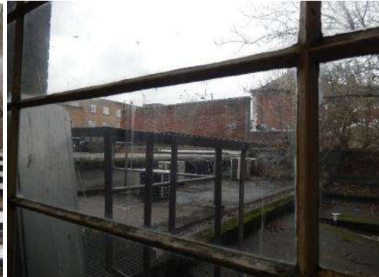
View of the Site from the stairs looking across the shop unit excluded from the local listing
