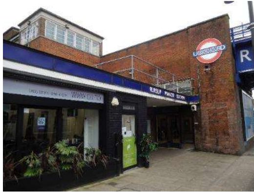
Northern entrance to Station with doors in screen wall
