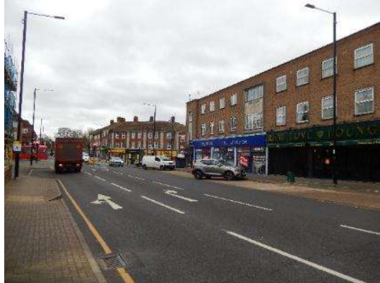
View east towards crossroads from Pembroke Rd
