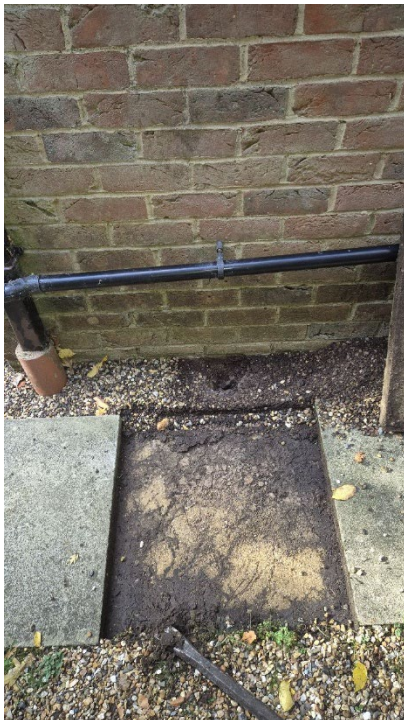
Photo 3 (Showing TP3 moved)
