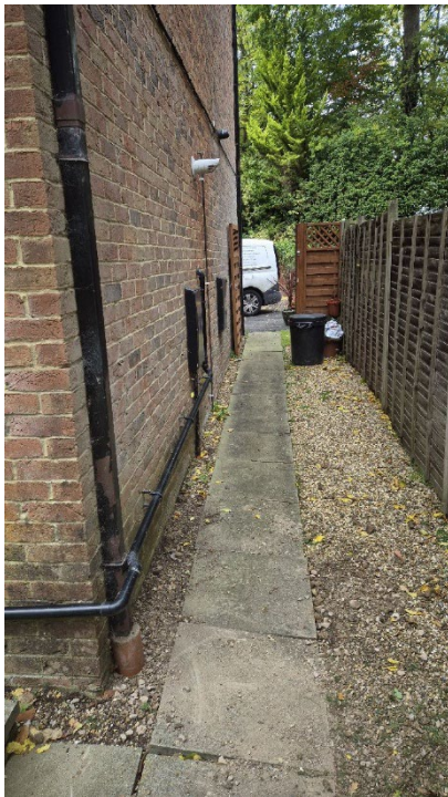
Photo 11 (Showing RWP 6 & RWP7)
