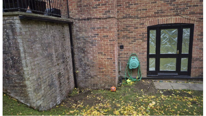
Photo 10 (Showing RWP5 & FWG1)
