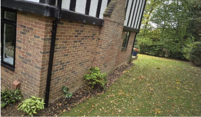
Photo 9 (Showing RWP3 & RWP4)
