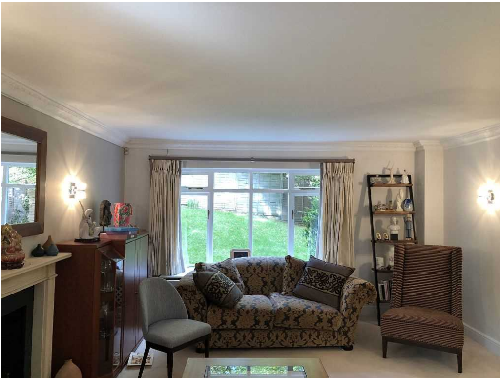
Ground floor right side through lounge. Cracks mainly around windows to front and back elevation
