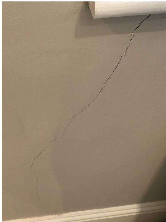
Front elevation second floor bedroom above garage. Bottom right corner crack 1mm jagged
