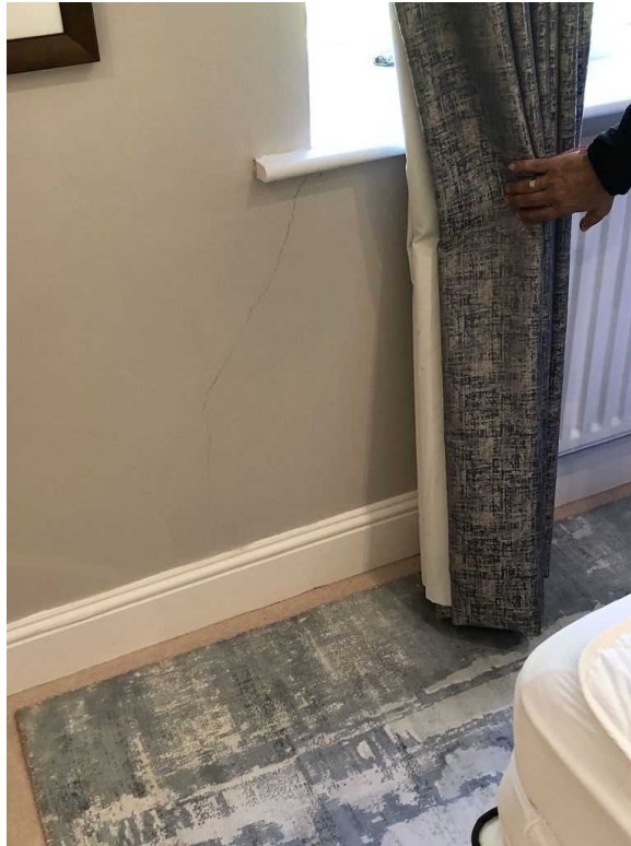
Front elevation second floor bedroom above garage. Bottom right corner crack 1mm jagged
