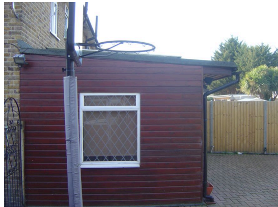
Existing rear extension
