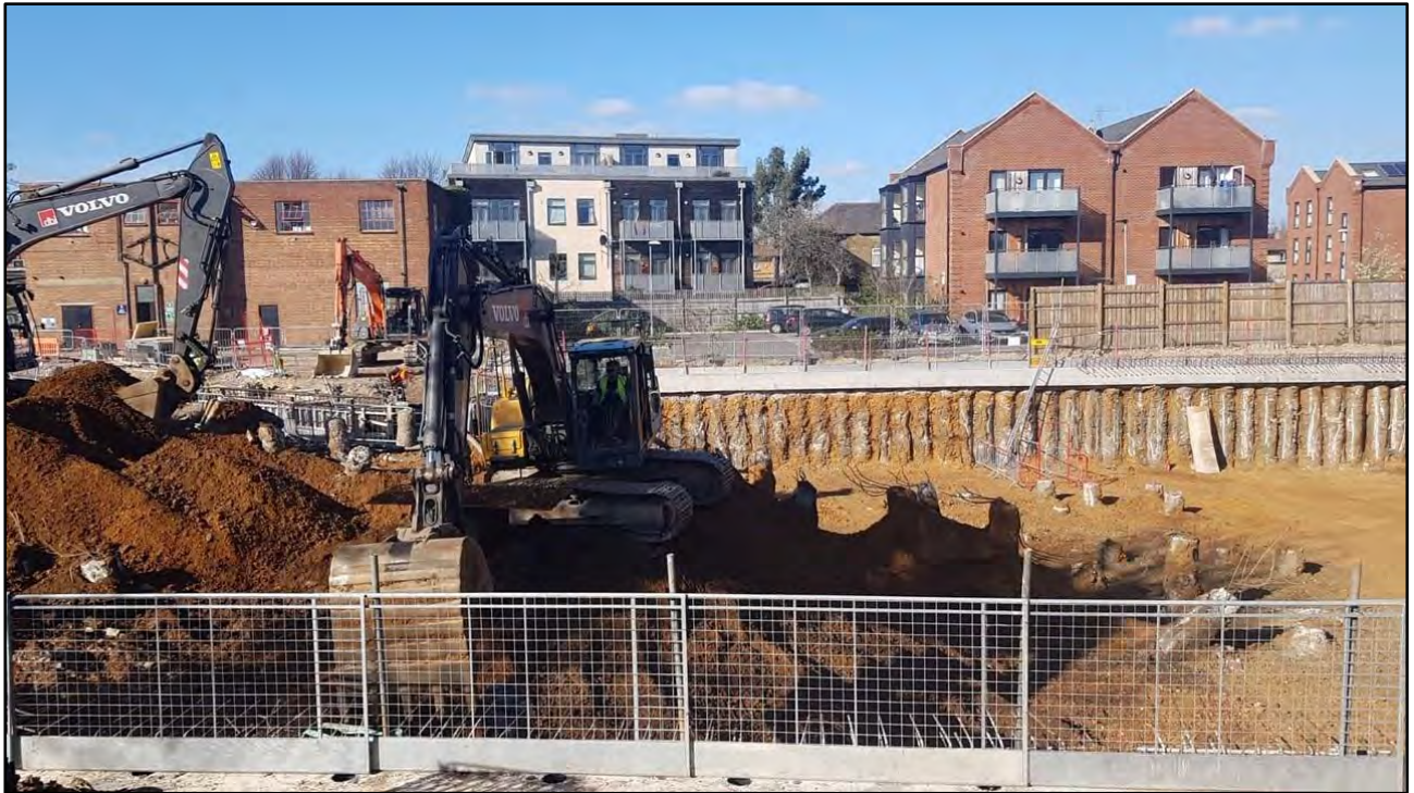
Plate 2 Basement excavation looking roughly north
