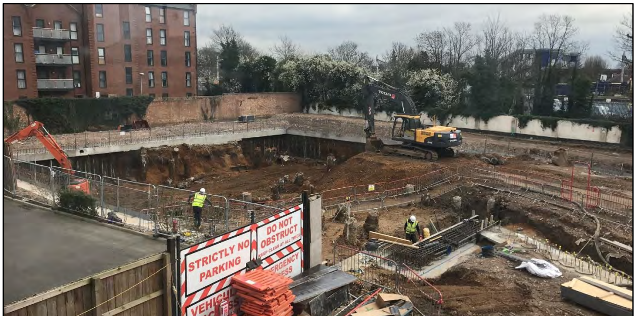
Plate 1 Basement excavation looking rough south east
