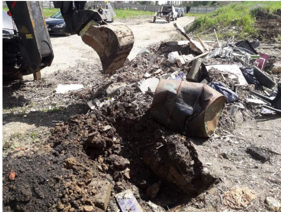
PHOTO 15: FFTP102 with respect to the empty steel barrel.
