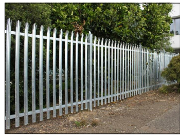
3. PALISADE FENCING TO PLANT AREA
