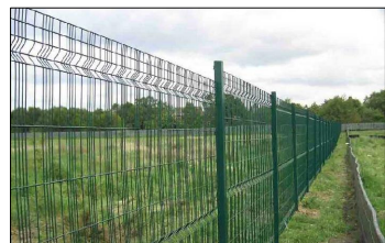
2. METAL SECURITY FENCE ALONG FRONT
