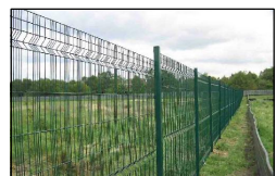
2. METAL SECURITY FENCE ALONG FRONT
