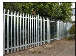
3. PALISADE FENCING TO PLANT AREA
