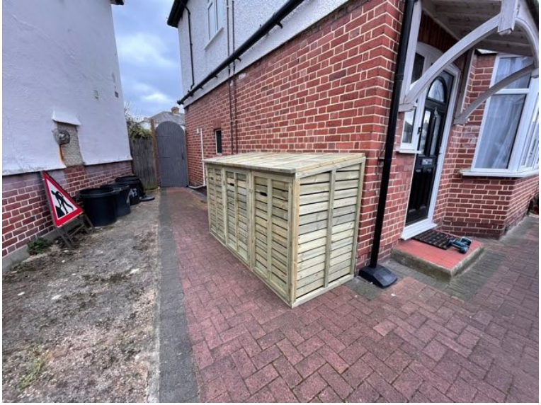
1. Photo of the bin store measuring 2290W x 850D x 1290H (mm) annotated on the site plan.
