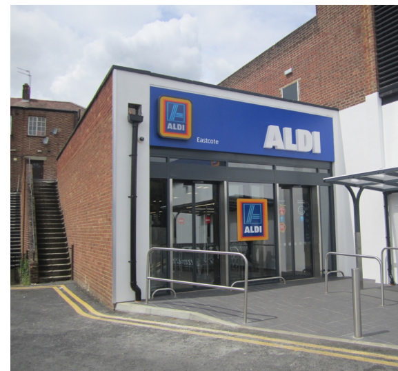
Rear side view of 127-133 Field End Road, Hillingdon
