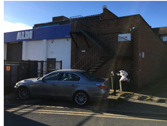
Rear view of 127-133 Field End Road, Hillingdon
