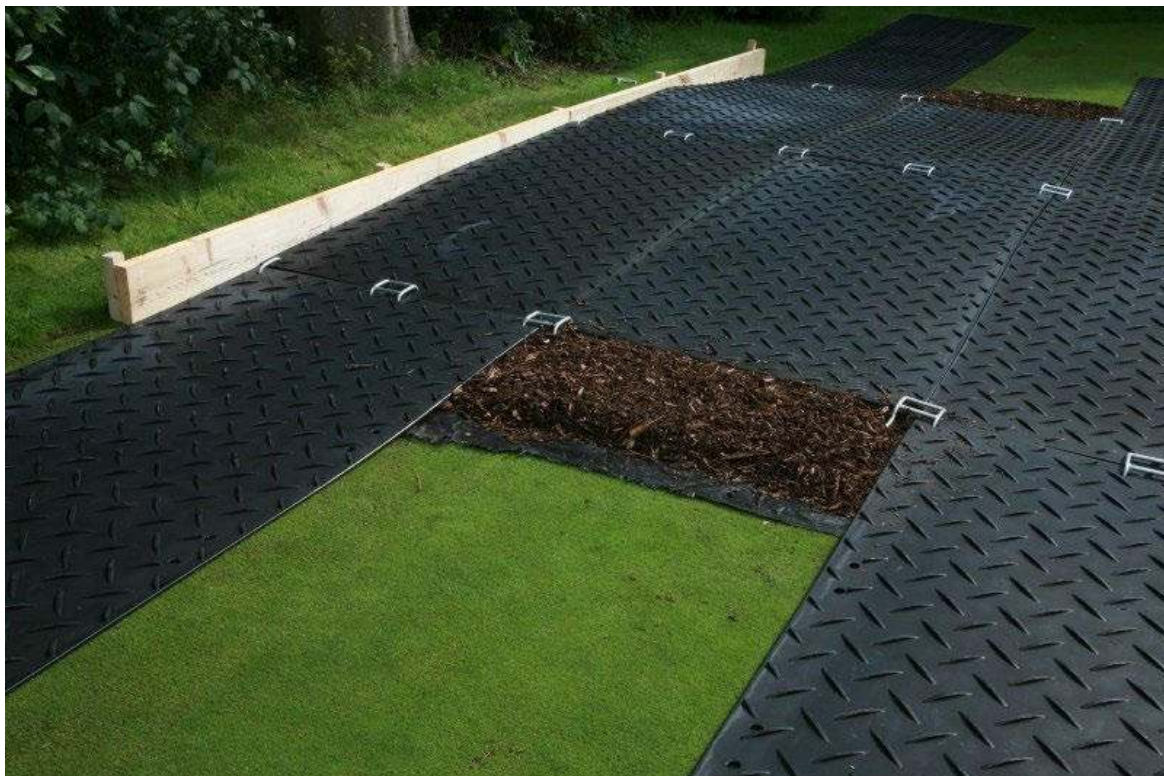
Figure 1. Example of propriety inter-linked ground protection boards placed on top of a compression-resistant layer (e.g. 150 mm depth of woodchip), laid onto a geotextile membrane, suitable for pedestrian-operated plant up to a gross weight of 2 t
