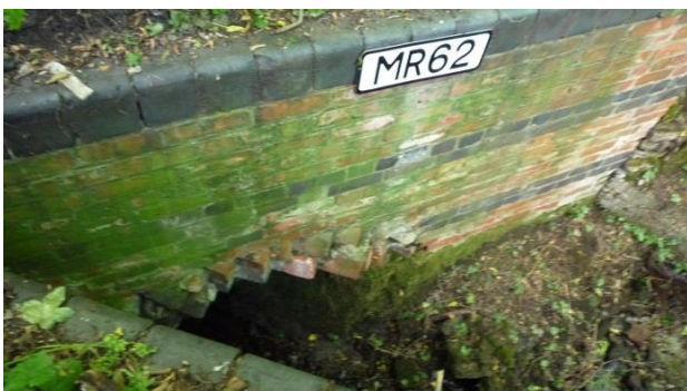
Figure 3—4 Headwall at upstream end of railway culvert
