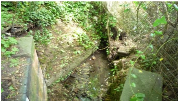
Figure 3—4 Headwall at upstream end of railway culvert
