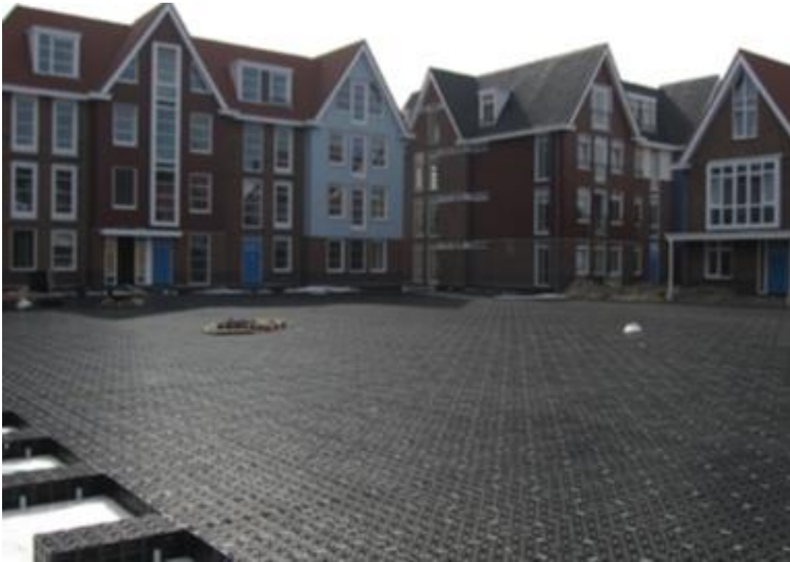
Figure 5—2: Permeable paving to car parking areas with geo-cellular units under to attenuate surface flows and roof drainage
