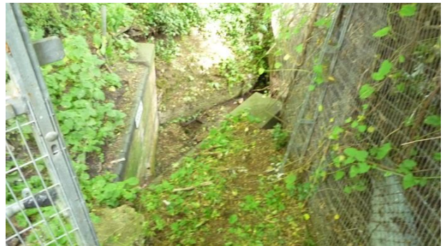
Figure 3—3 Open ditch at entrance to culvert
