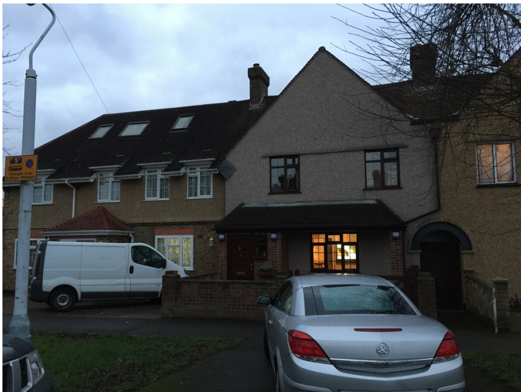
Figure 2 - No.6 and No.8 Peach Tree Avenue
