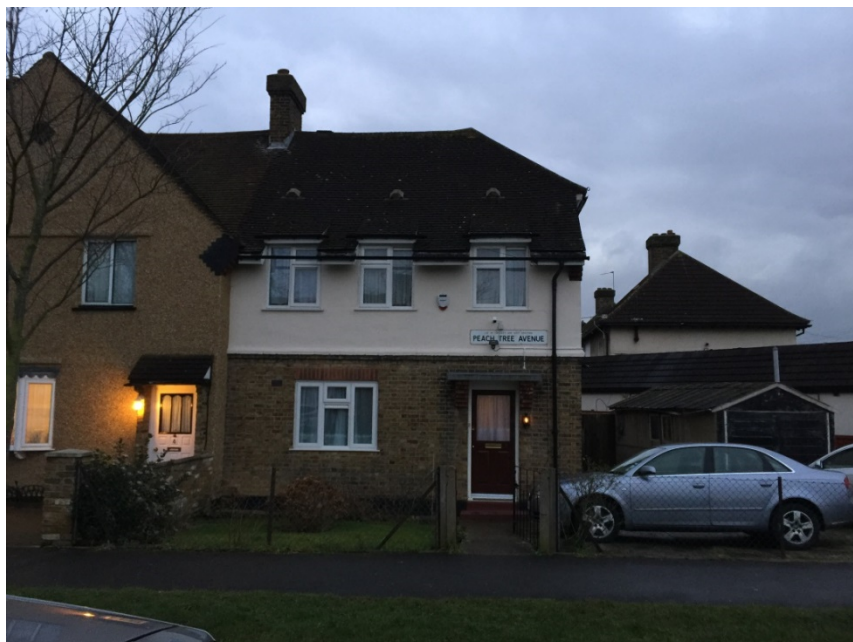
Figure 5 – Existing Front Elevation of the property
