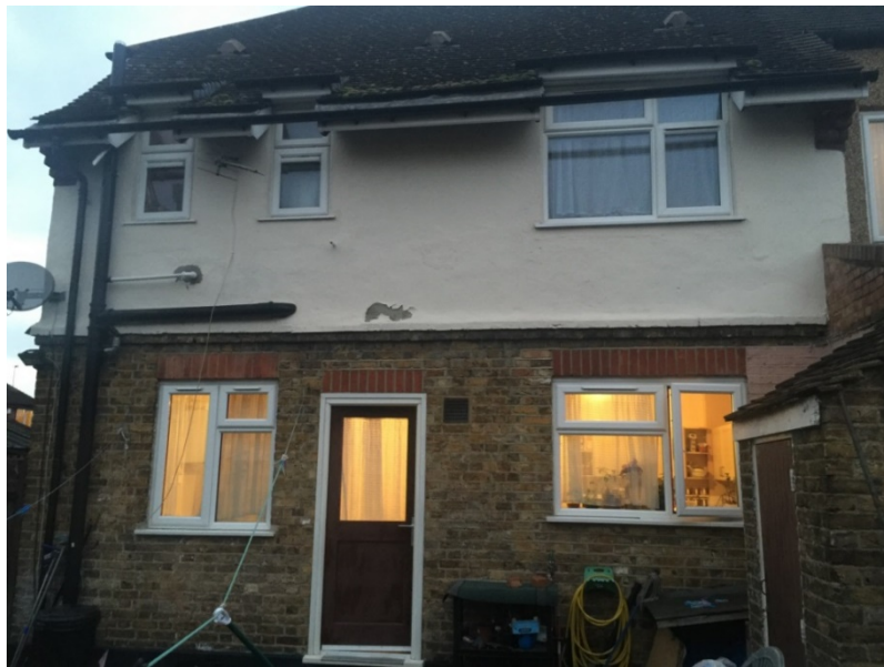
Figure 4 – Existing Rear Elevation of the property.
