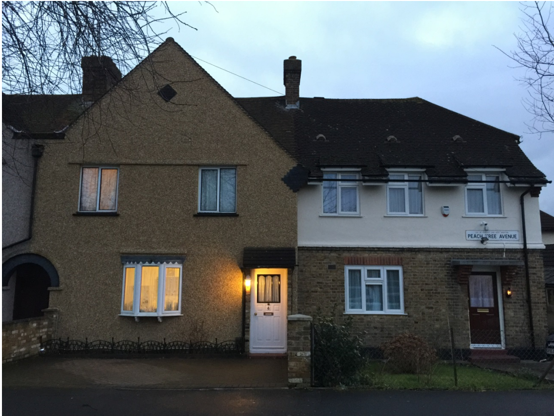
Figure 1 - No.2 and No.4 Peach Tree Avenue
