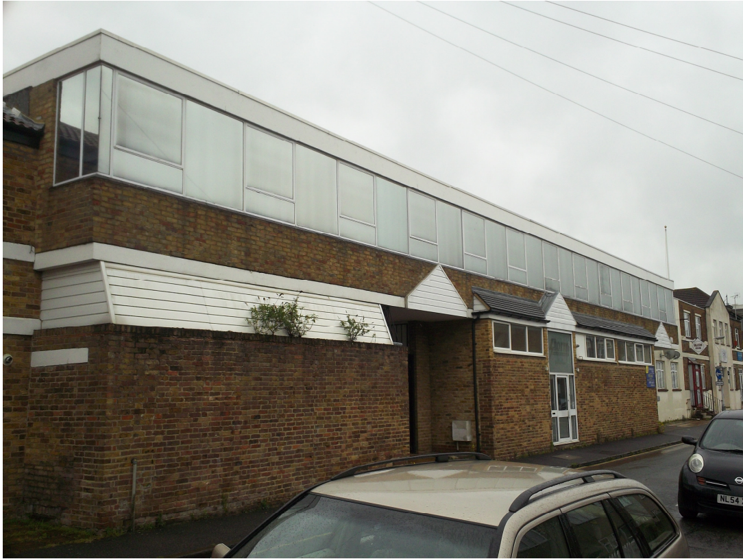
PHOTO 1: 12-14 BENTINCK COURT TAKEN FROM BENTINCK ROAD
