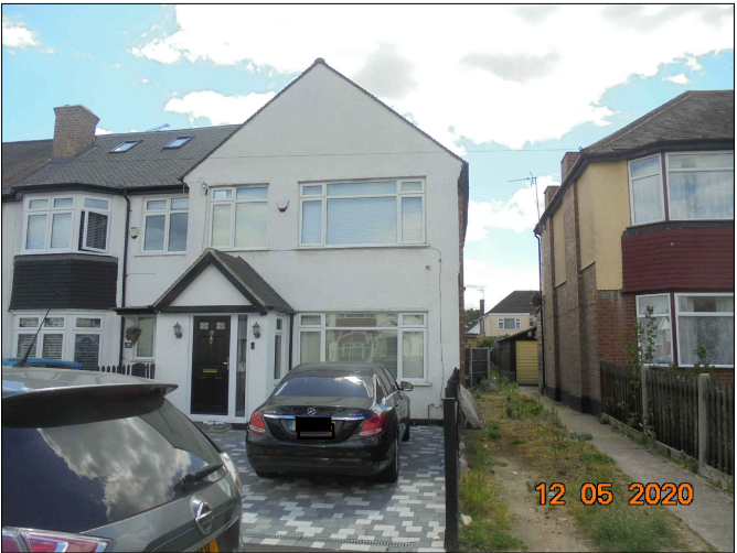
Existing Front Elevation Photograph
