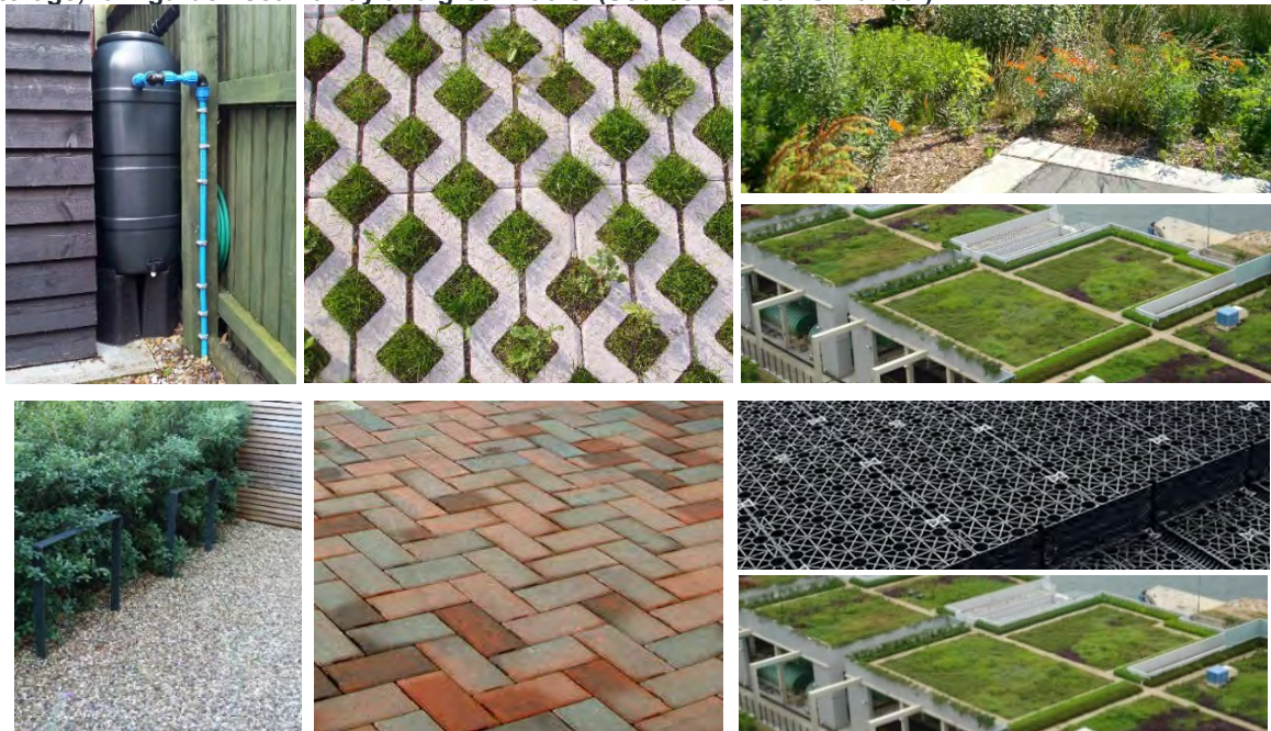
Figure 2 Surface water storage facilities and potential SuDS features – rainwater harvesting, on-site tank storage, rain garden soak-away and green roofs. (Source: UK SuDS Manual).
