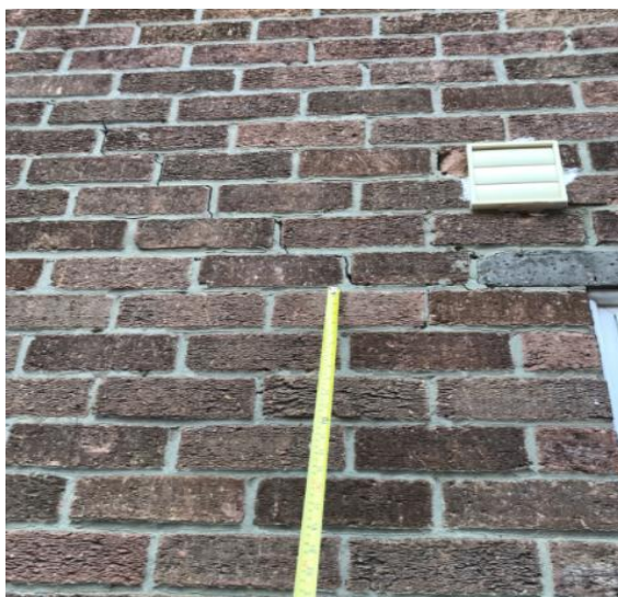
Flank wall cracking
