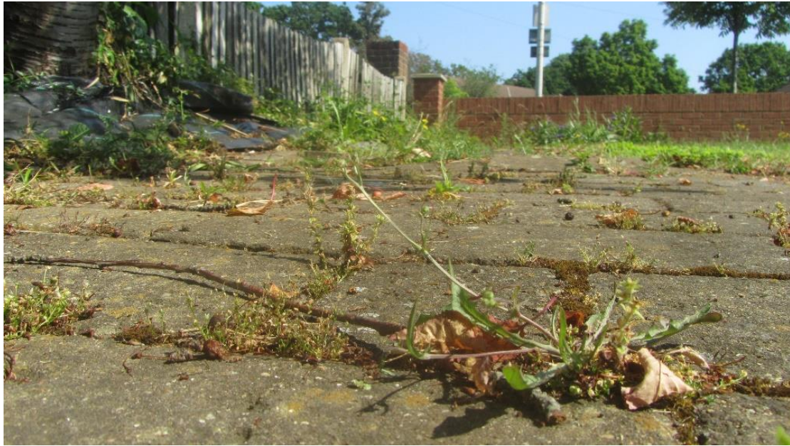
PHOTOGRAPH NO. 7 – upheaved and disturbed surface of the driveway
