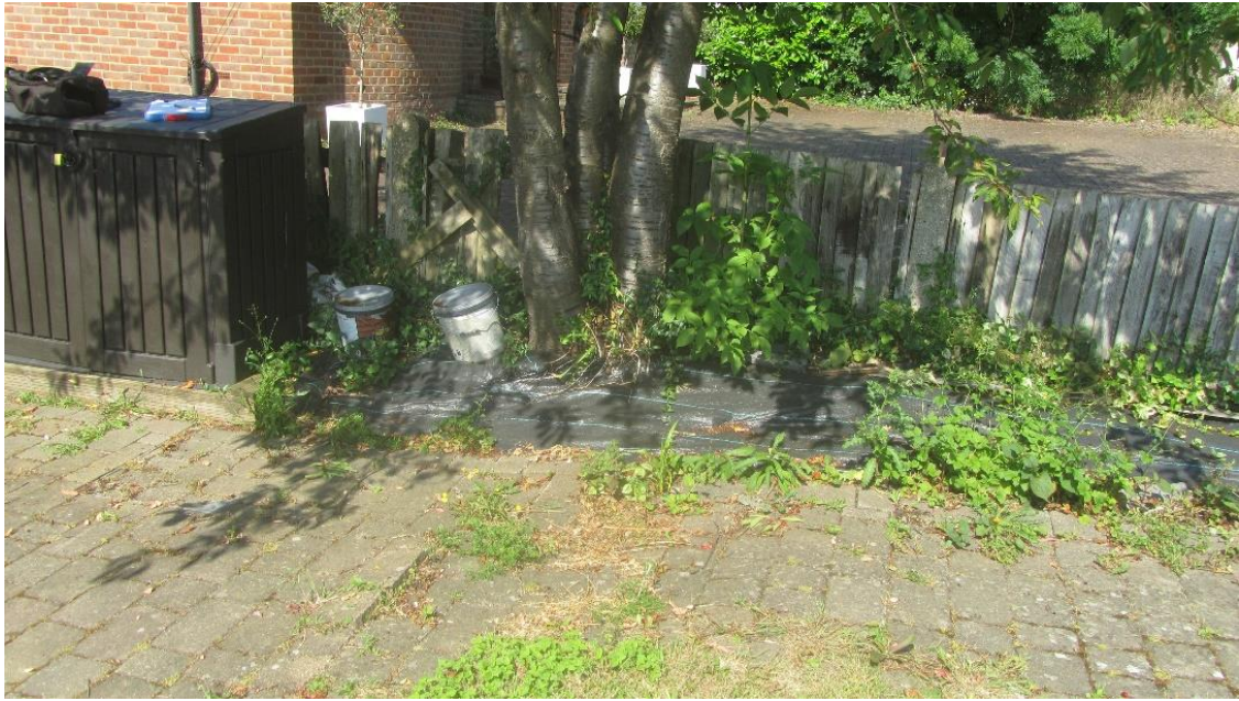
PHOTOGRAPH NO. 3 – base of T1 with visible uplift of the nearby pavements
