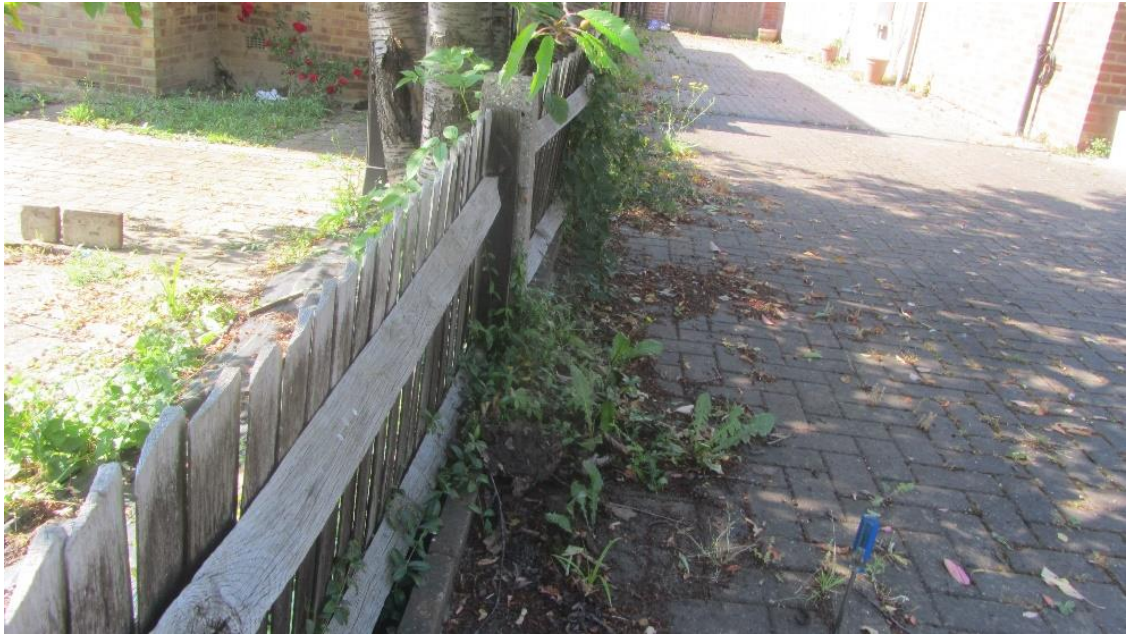
PHOTOGRAPH NO. 11 – uplift of the driveway of No. 18 – likely due to tree root growth
