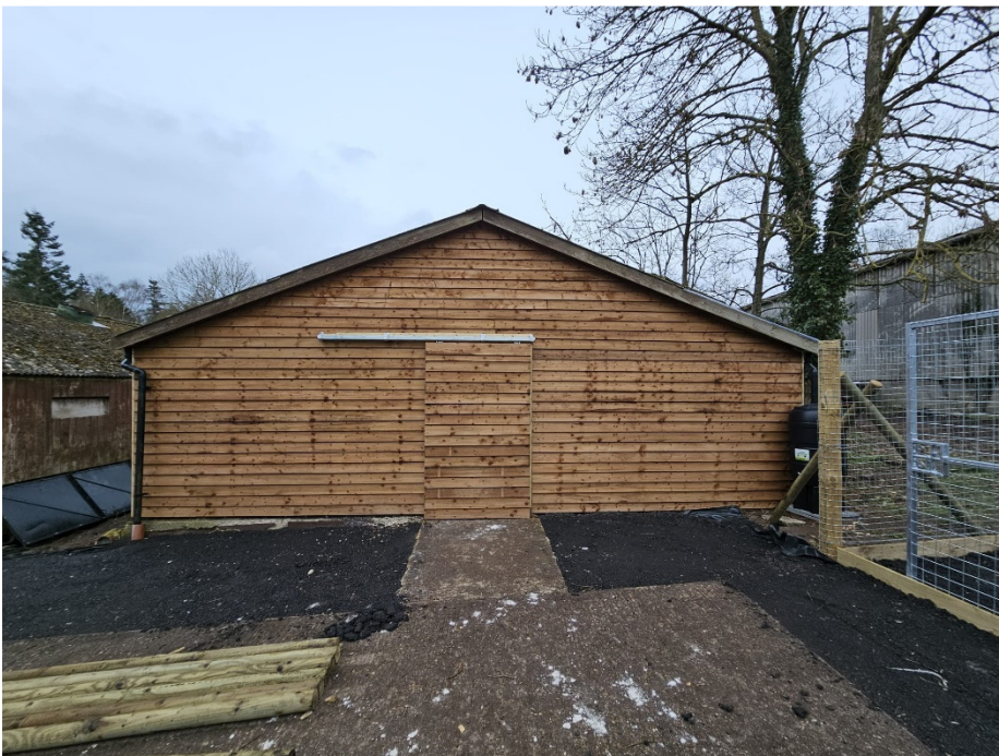
Photo 5 – External Barn two and three with new timber cladding to match existing.
