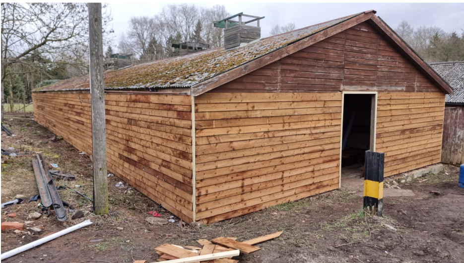
Photo 6 – External Barn two and three with new timber cladding to match existing.
