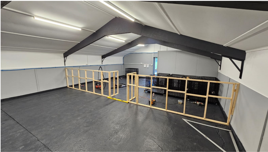
Photo 3 – Inside of Barn 2 and 3. New concrete floor and lighting.
