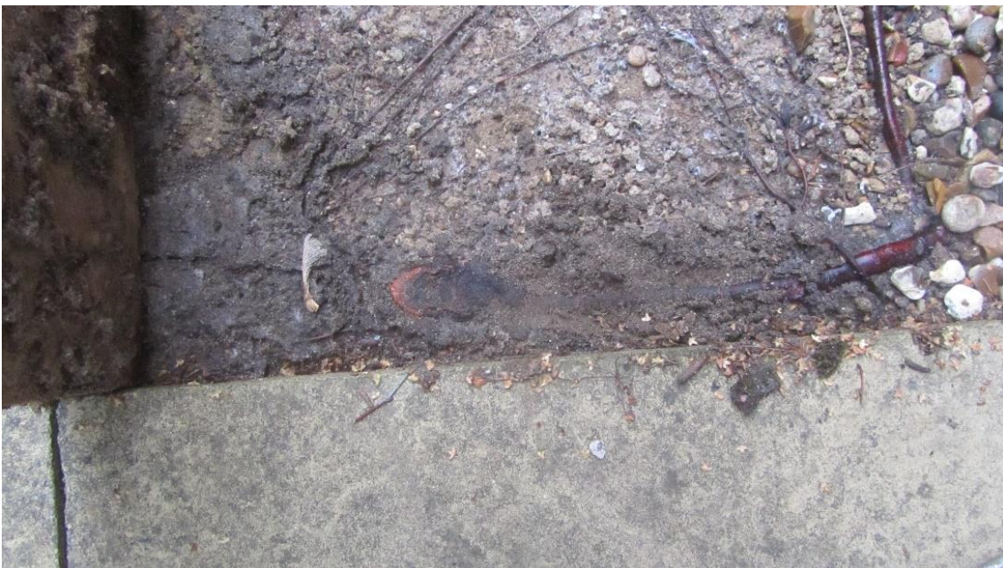
PHOTOGRAPH NO. 14 - T3 – BIRCH TREE ROOTS IN SIDE PASSAGEWAY BY EASTERN FLANK WALL
