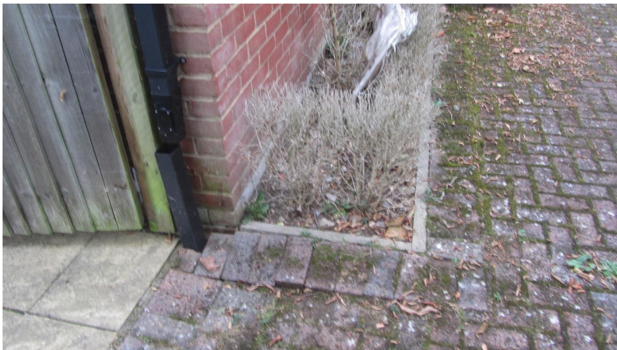
PHOTOGRAPH NO. 8 - DISTURBED DOWN-PIPE AND BLOCK PAVING BY SOUTHWESTERN CORNER OF THE DWELLING HOUSE
