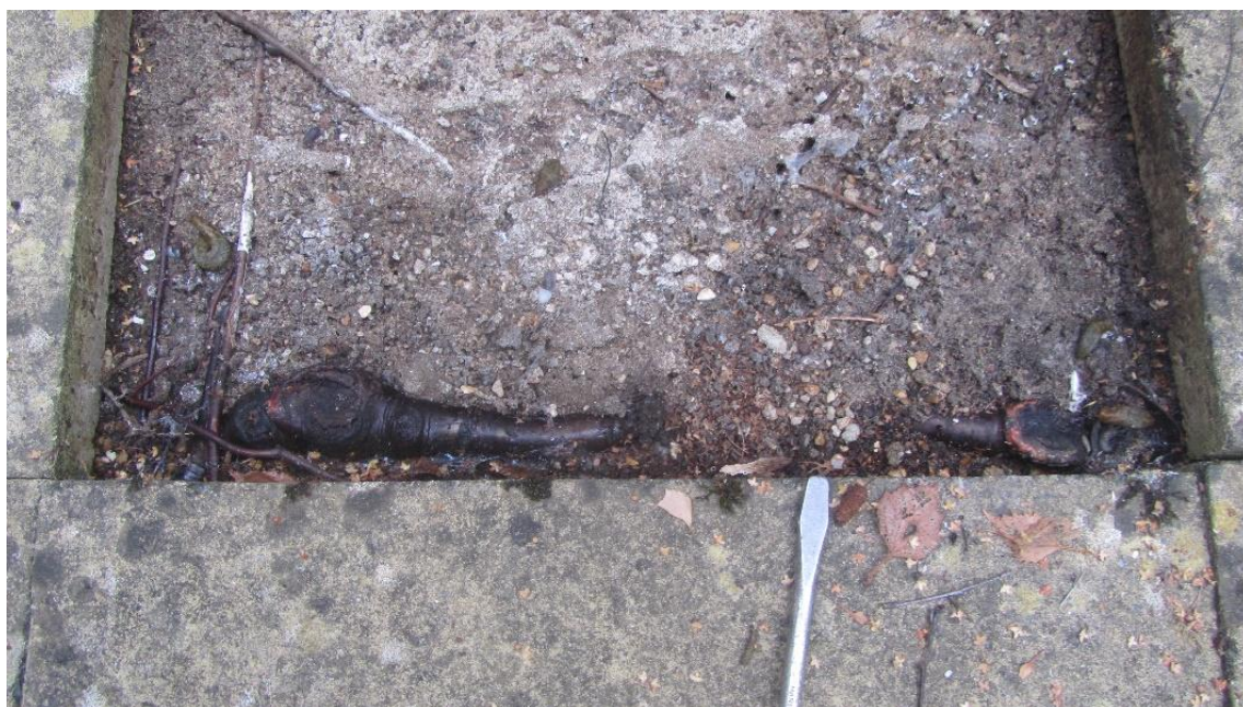
PHOTOGRAPH NO. 12 - T3 – BIRCH TREE ROOTS IN DISTAL CORNER OF PAVED AREA NEAREST THE TREE AND 2.5 M FROM BOUNDARY WITH NO. 2 ELMSDENE MEWS
