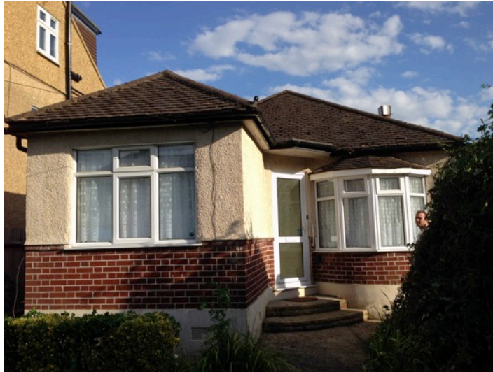
Photograph 4: Front view of the bungalow.
