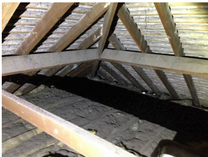
Photograph 7: View of roof space.
