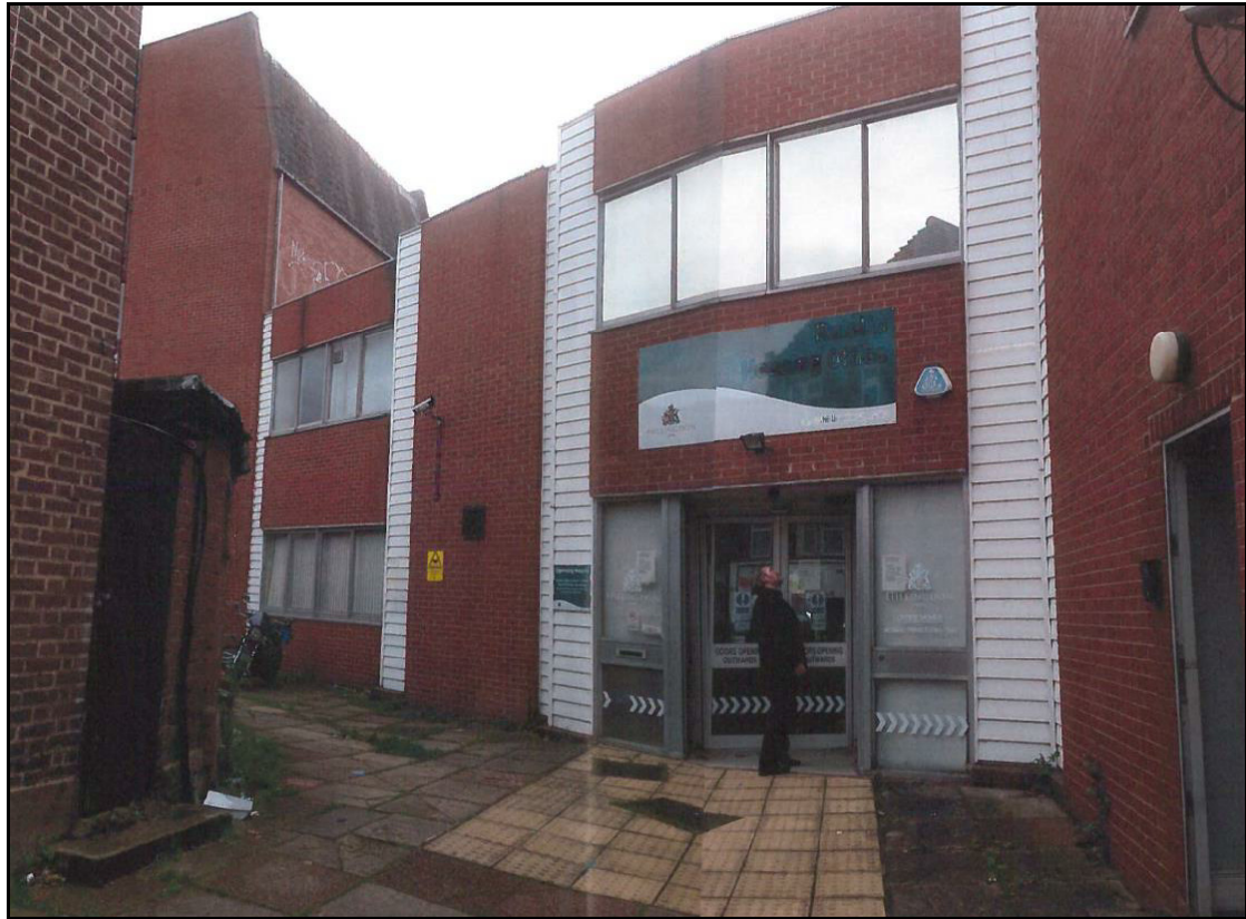
Figure 2: Photograph of Front Entrance to Existing Building
