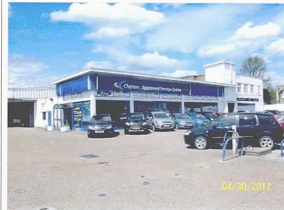
Demolition of Structures
