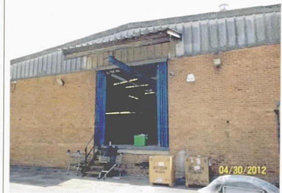
Works at Height
