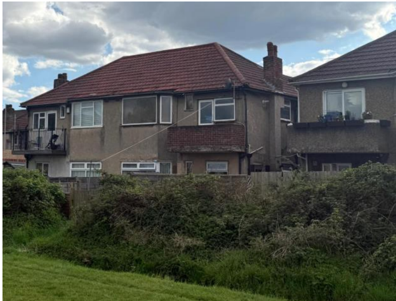
Figure 2: photo taken from the fields show that the balcony feature extends all along the row of adjacent houses, all the way to the end of the row
