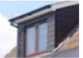
Catslide Dormer Window Plain tile to match roof tile
