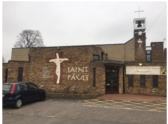
Existing main entrance (front side)
