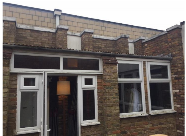
Existing rear entrance
