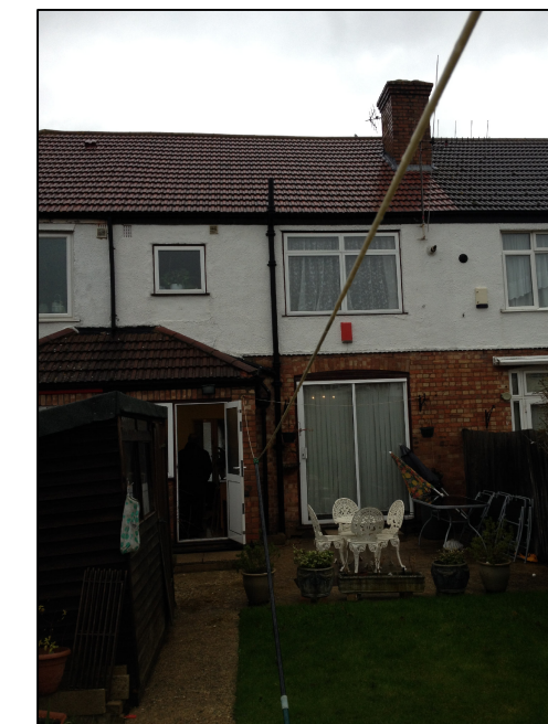
PHOTOGRAPH REAR ELEVATION
