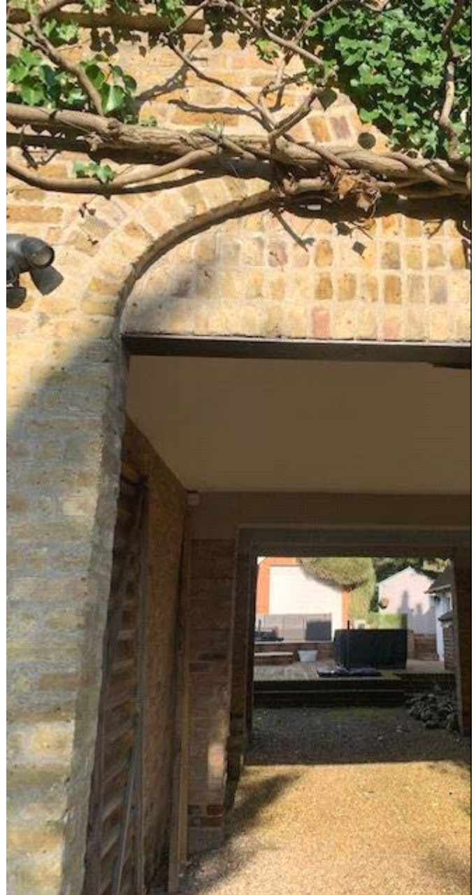
Example of arch above entrance to the garage
