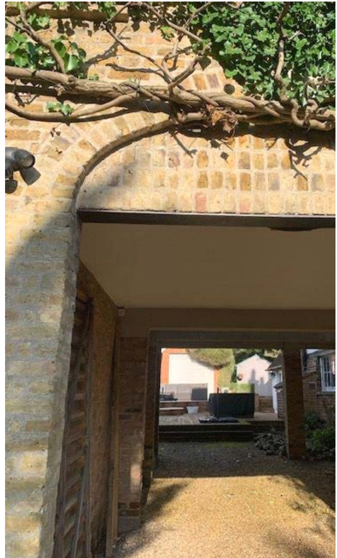
Arch above garage doors
