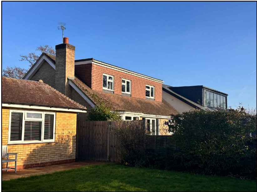
REAR /SIDE VIEW OF NO. 30
