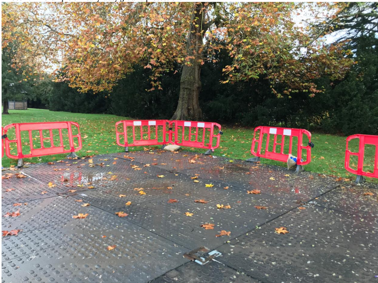
Photo 2. An example of heavy-duty ground protection.
