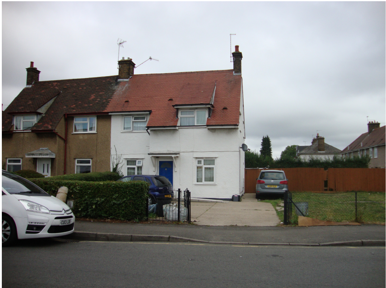
EXISTING BUILDING ON SITE
