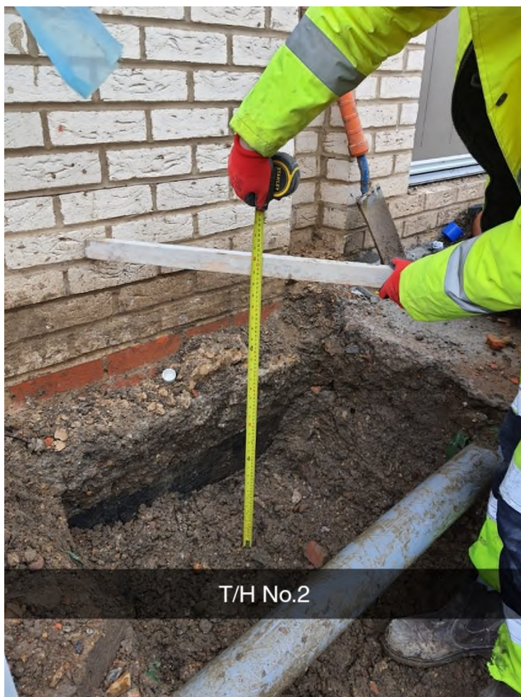
Plate 3: Plot 2 shrub planting area measurement (Provided by Bellway).
