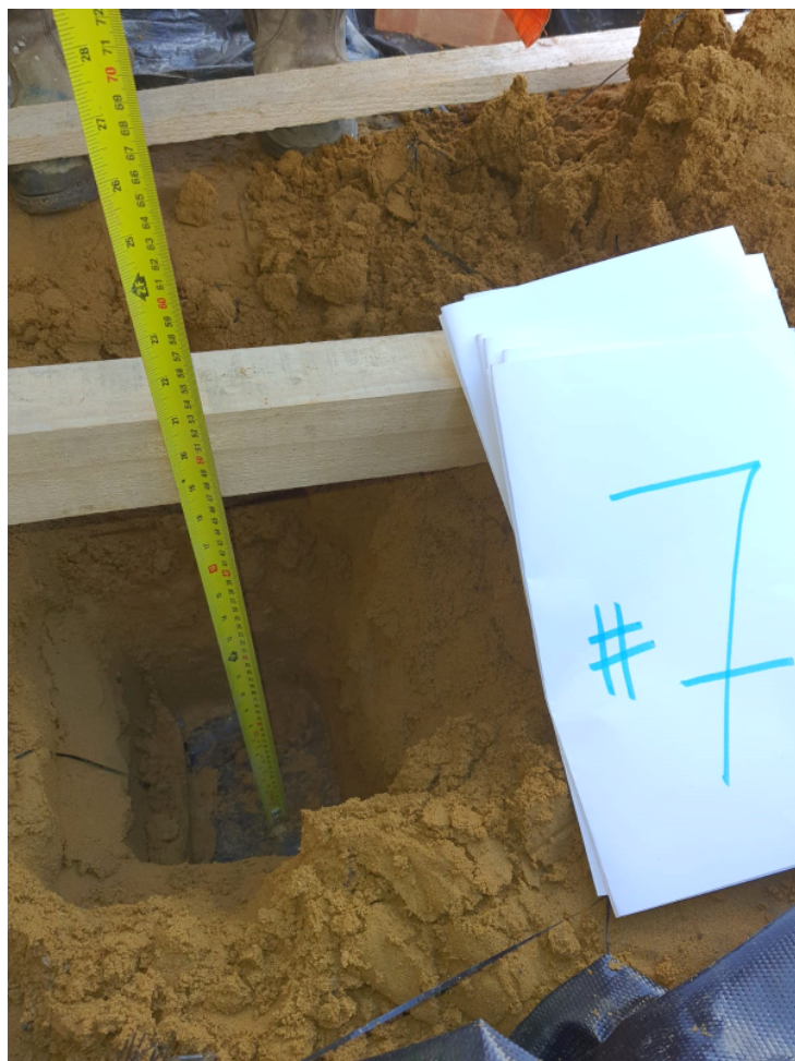
Plate 14: Plot 7 hand dug pit with thickness of subsoils indicated (Provided by Bellway)
