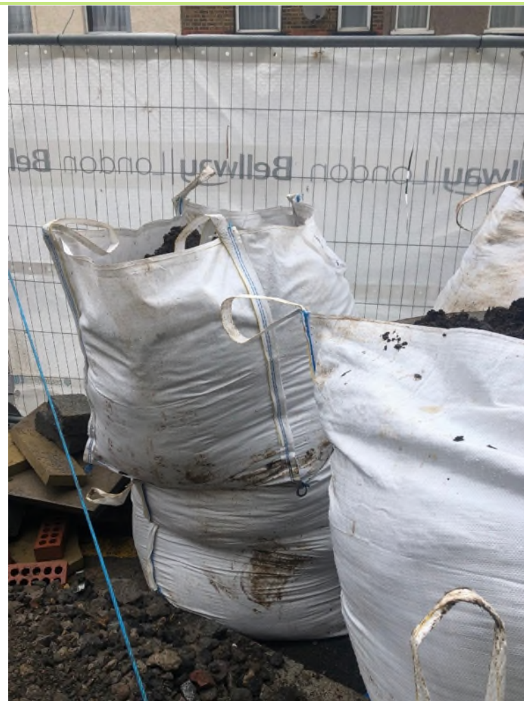
Plate 18: Topsoil bulk bag 3 from which a sample was taken for analysis (Taken by LEAP Engineer).
