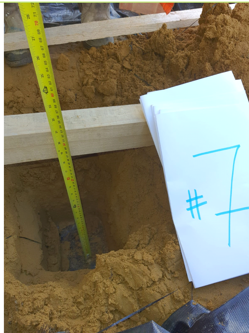
Plate 16: Plot 7 hand dug pit with thickness of subsoils indicated and geotextile membrane visible (Provided by Bellway).
