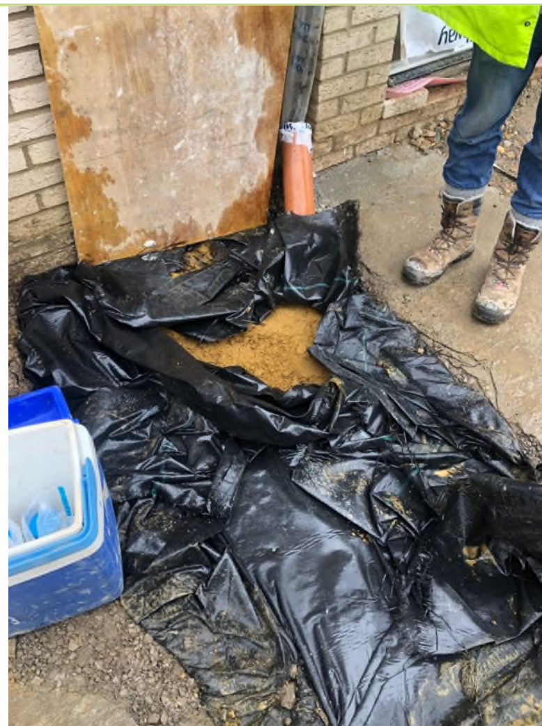
Plate 10: Plot 4 with geotextile wrap around subsoil within shrub planting area (Taken by LEAP Engineer).
